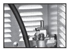
Remove the steel plug from the number one outlet port and the brass fitting for the fuel hose from the number two port.
